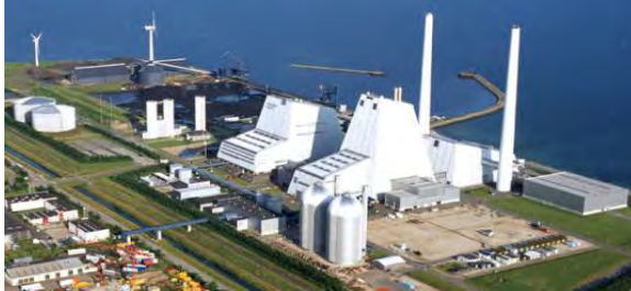
Avedøre II (2001) / DONG Energy A/S CHP / 485 MWe & 545 MJ/s heat
