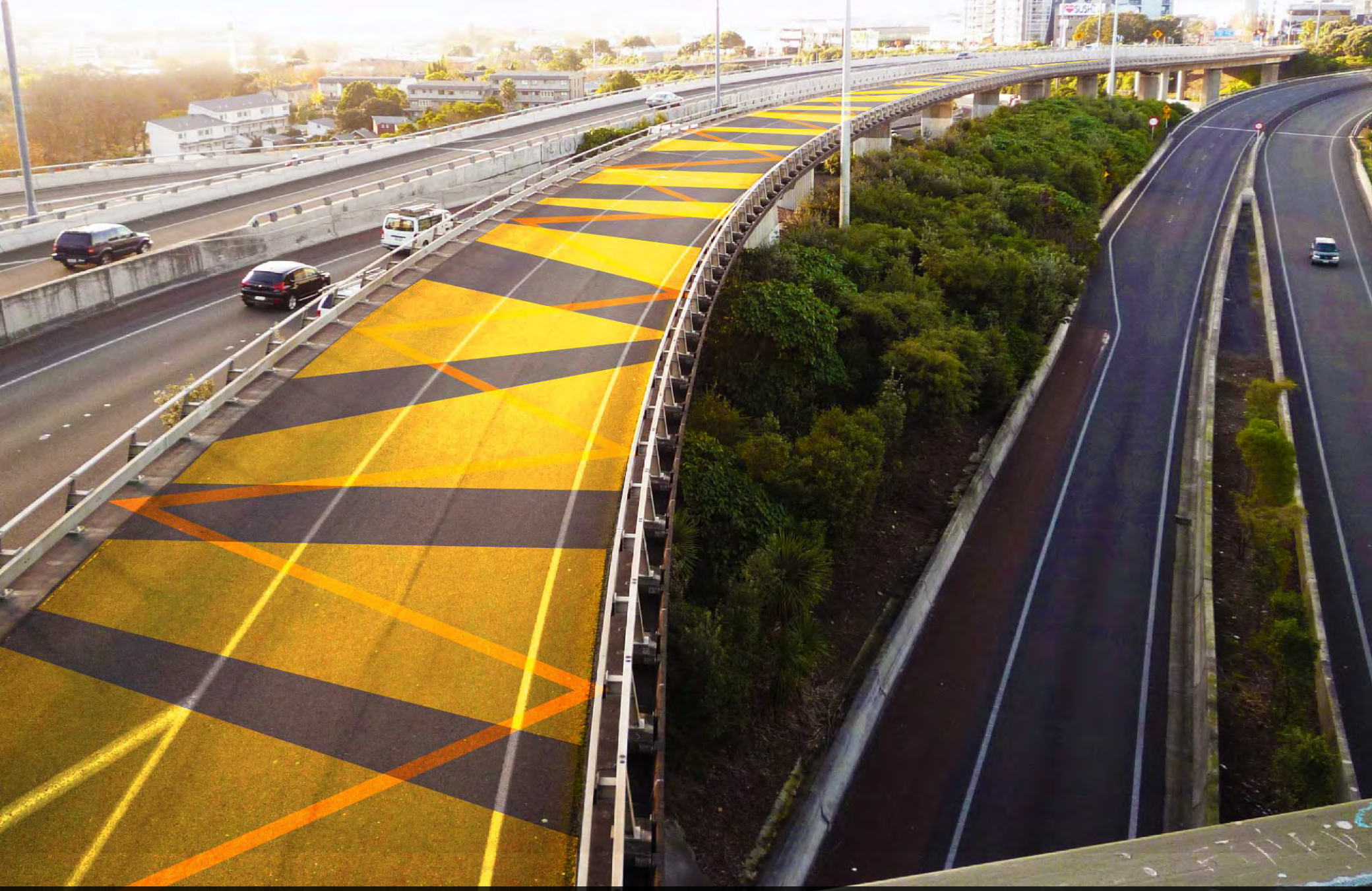
Old Nelson Street off ramp - Potential
