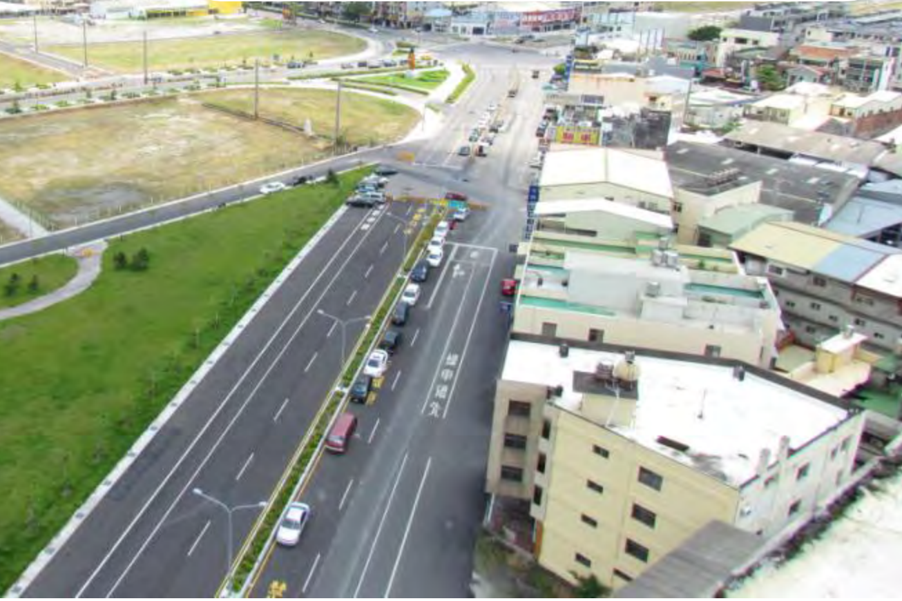
The Railway Elevation Project in Yuanlin
