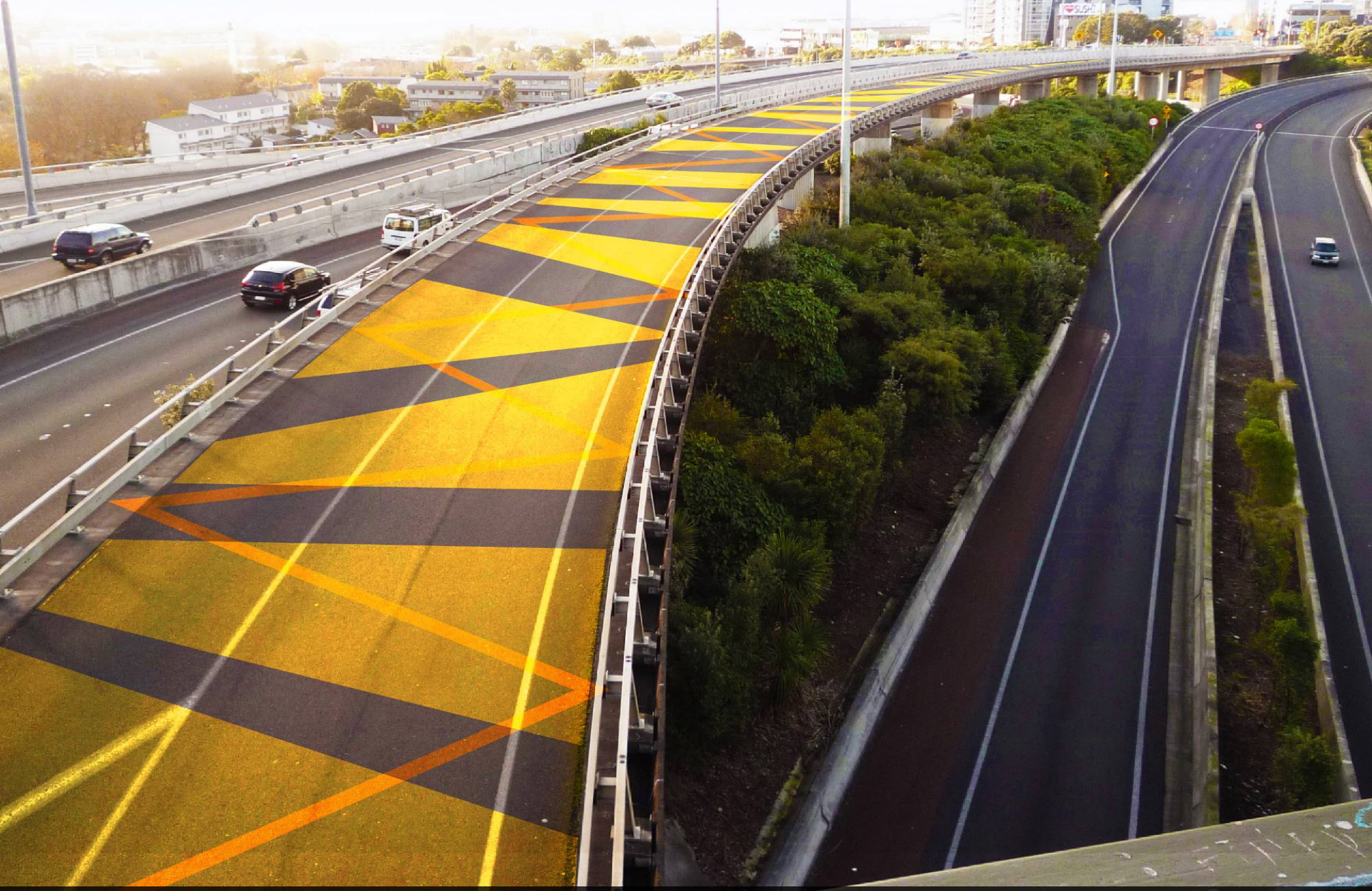
Old Nelson Street off ramp - Potential
