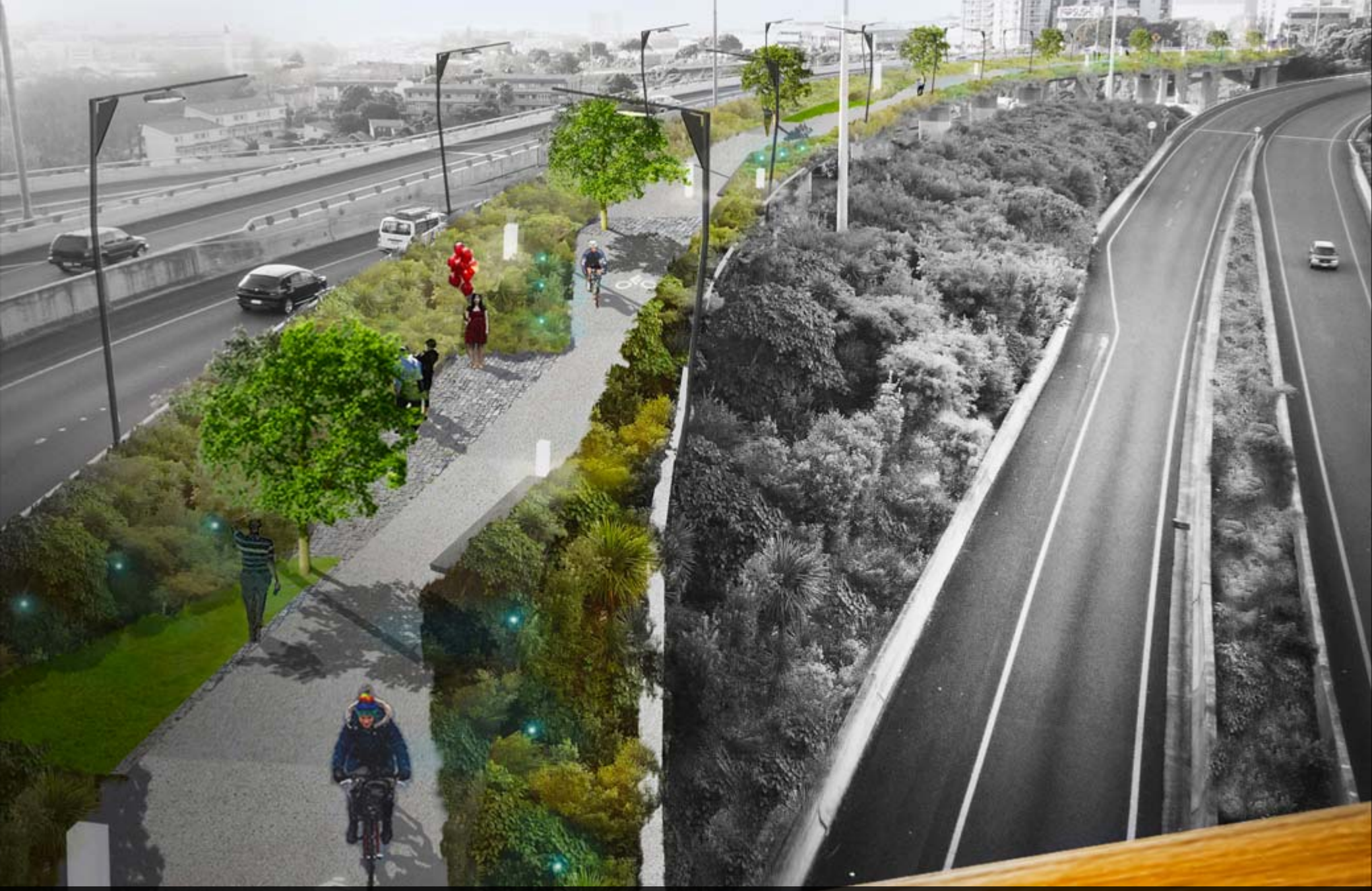
Old Nelson Street off ramp - Potential
